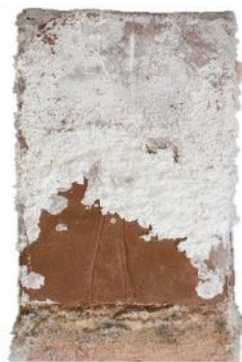
Front view of brick
